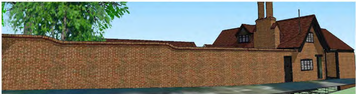
View from west existing
