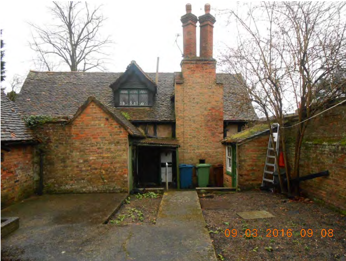
FLANK ELEVATION OF COTTAGE FROM RAISED PATIO
