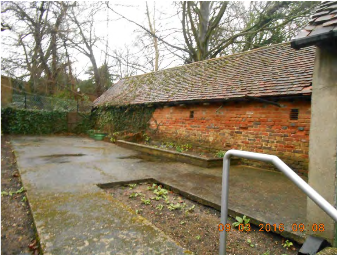
EXISTING COWSHED VIEWED FROM WITHIN PATIO AREA
